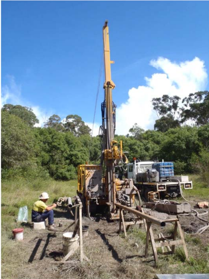
Figure 1: Rotary core drilling of monitoring bore GW04
