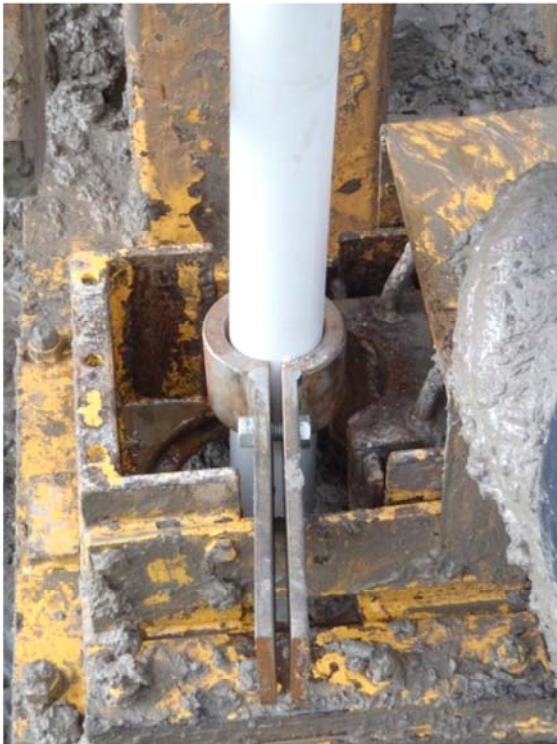
Figure 2: Monitoring bore installation using clamp
