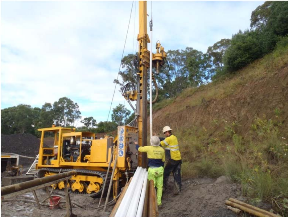
Figure 3: Monitoring bore installation using hoist plug on GW03
