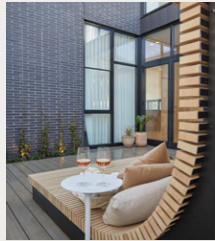
Luke & Jasmin's Back Garden. Nero Linear, Morada. Bond pattern: Stretcher. Mortar: Grey. Joint: Raked.
