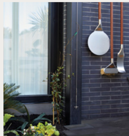
Luke & Jasmin's Back Garden. Nero Linear, Morada. Bond pattern: Stretcher. Mortar: Grey. Joint: Raked.
