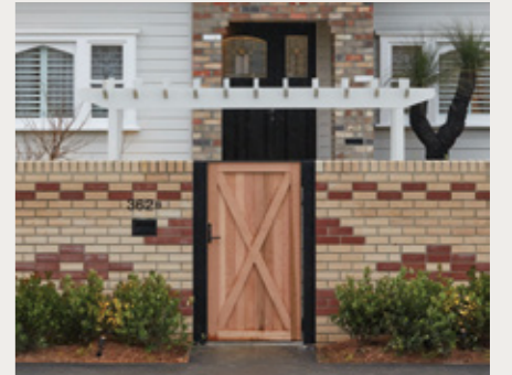
Sarah & George's Brick Fencing. McGarvie Red & Organic White, Dry Pressed Architectural. Bond patterns: Soldier Course Headers / Stretcher / Contrasting Colour Brick Feature. Mortar: Off-White. Joint: Round / Ironed.
