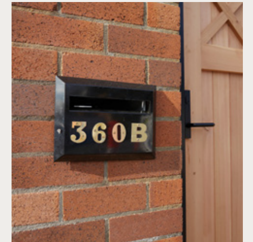
Luke & Jasmin's Brick Fencing. Black Beauty & Hawkesbury Bronze, Dry Pressed Architectural. Bond pattern: Stretcher Bond Wall & Piers. Mortar: Off-White. Joint: Round / Ironed.
