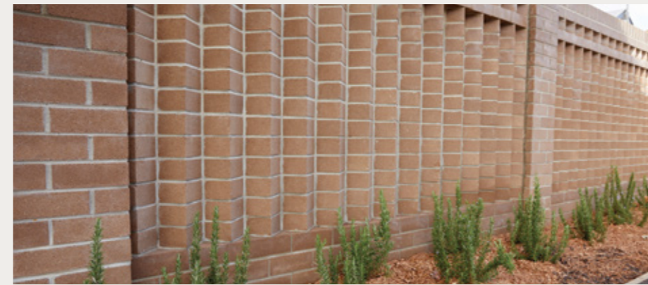
Megalong Valley Grey , Dry Pressed Architectural. Bond patterns: Soldier Course / Corbel Stack / Dog Tooth Brickwork / Stack Bond Piers. Mortar: Off-White. Joint: Round / Ironed.
